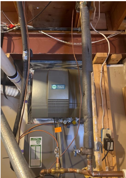
Furnace: Gas Burner
