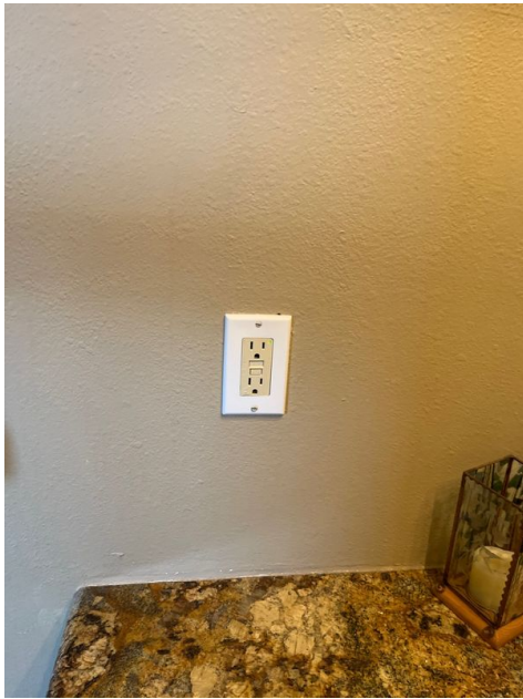
1st Floor Bathroom
